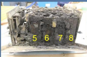
Substantial thermal damage
